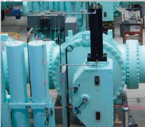
This butterfly valve is controlled by a  $\varnothing 10''$  actuator equipped with a  $\varnothing 3.5''$  high-strength stainless steel piston rod along with electronic feedback and banked accumulators
