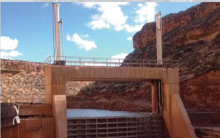
This spillway is operated by two Ø8" x 120" stroke, flange-mounted, mill-type actuators with a Ø4" high-strength, stainless steel piston rod, and protected from the outdoor elements by special paint.
