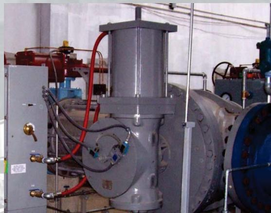
Ø18.00" actuator has a Ø4" stainless steel piston rod with a 4" stroke adjustment rod operates a Ø30" cone valve via a light hydraulic control panel.
